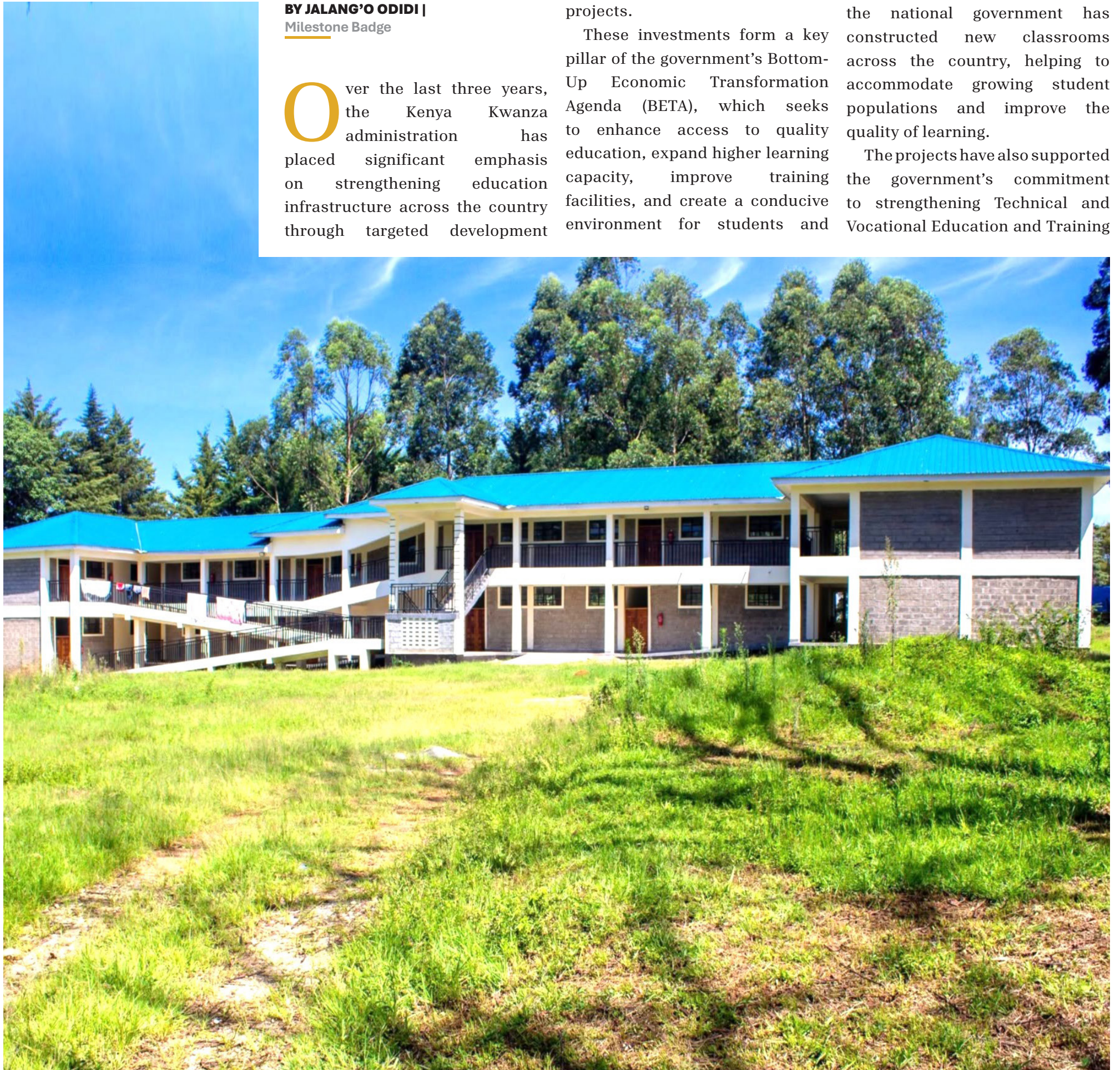
A section of the Eburngwe Technical and Vocational Centre in Vihiga County. PHOTO | Omboko Milemba.
