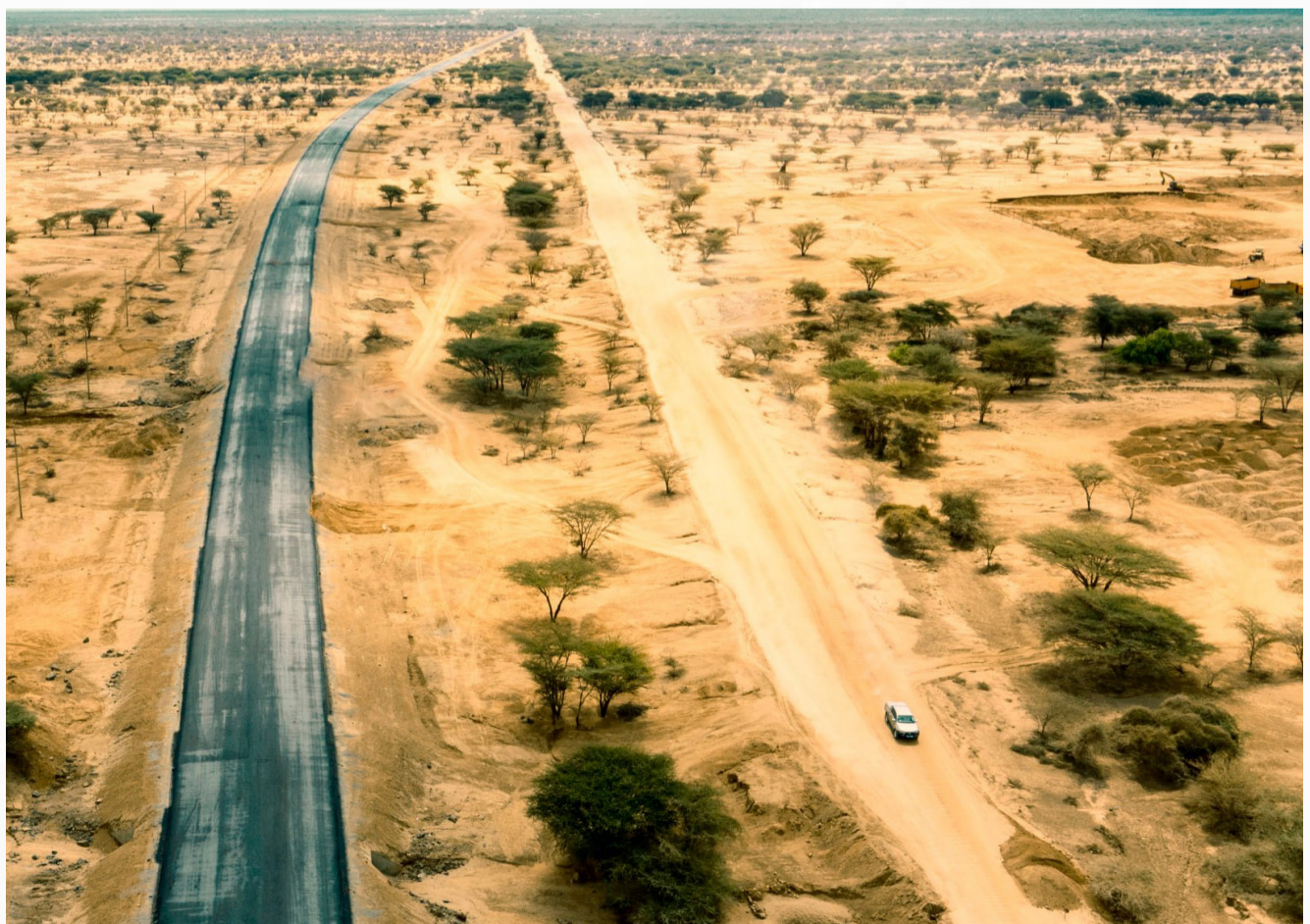
Section between Lokichar-Loichangamatak of the South Sudan Link Road. PHOTO | KeNHA
