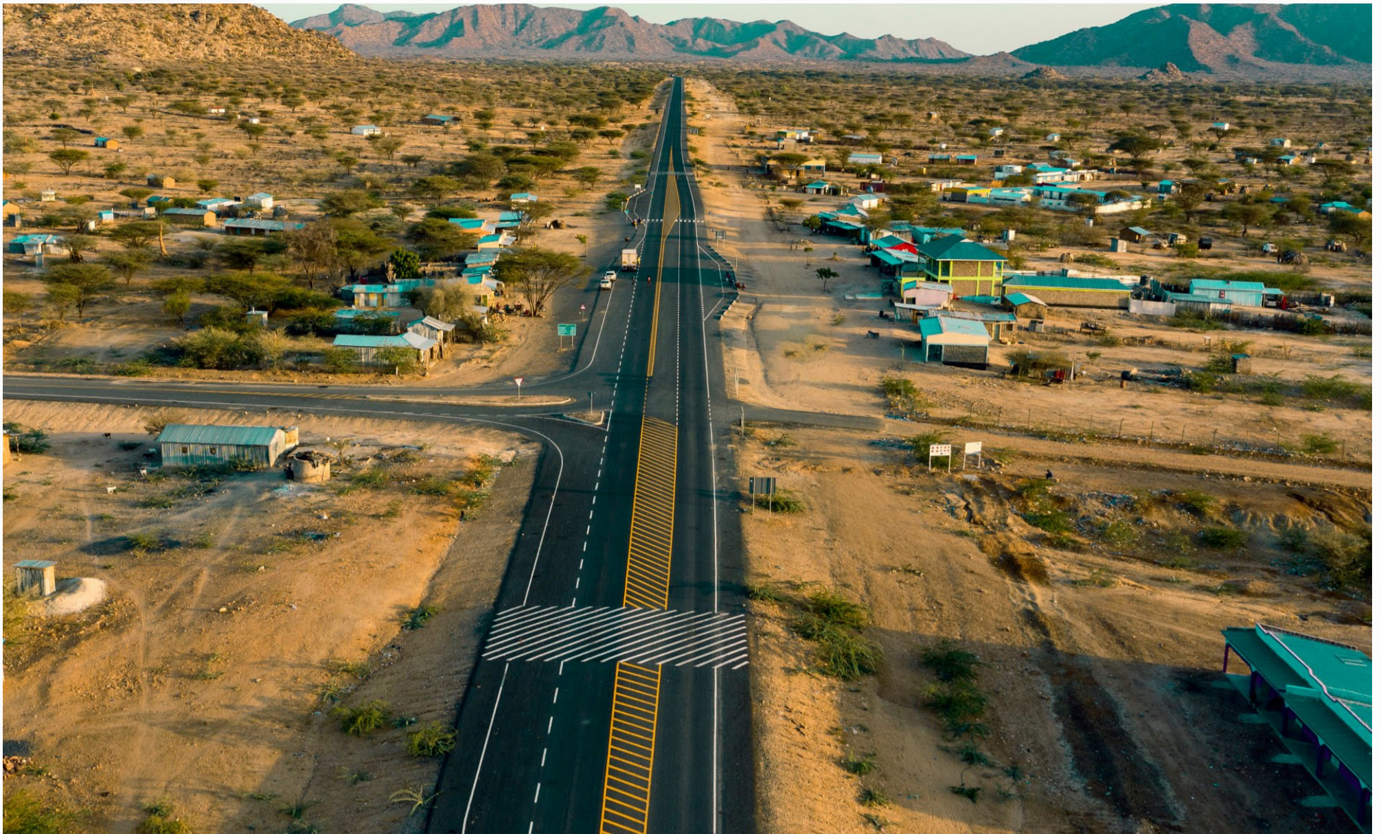
Makutano-Lokitaung Junction on the South Sudan link road. PHOTO | KeNHA
