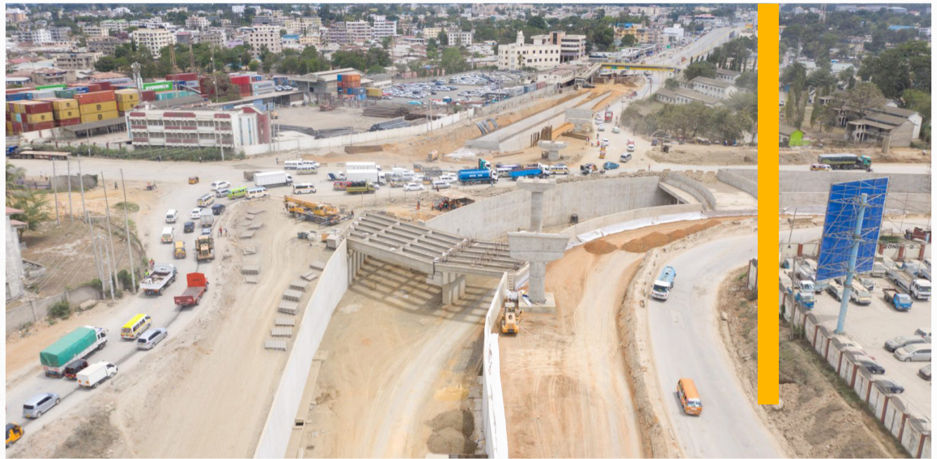
Construction of the Changamwe Interchange in Mombasa. PHOTO | KeNHA
