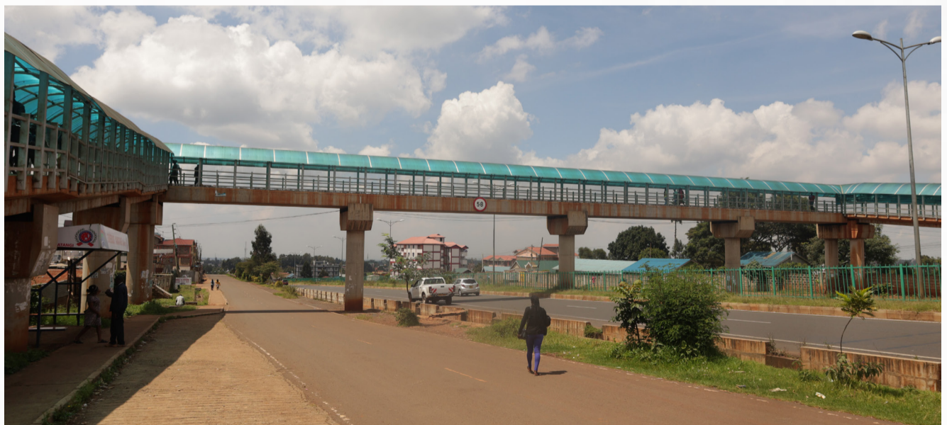
A foot bridge along Western bypass in Kiambu county on May 10,2026. PHOTO | Peter Obuya
