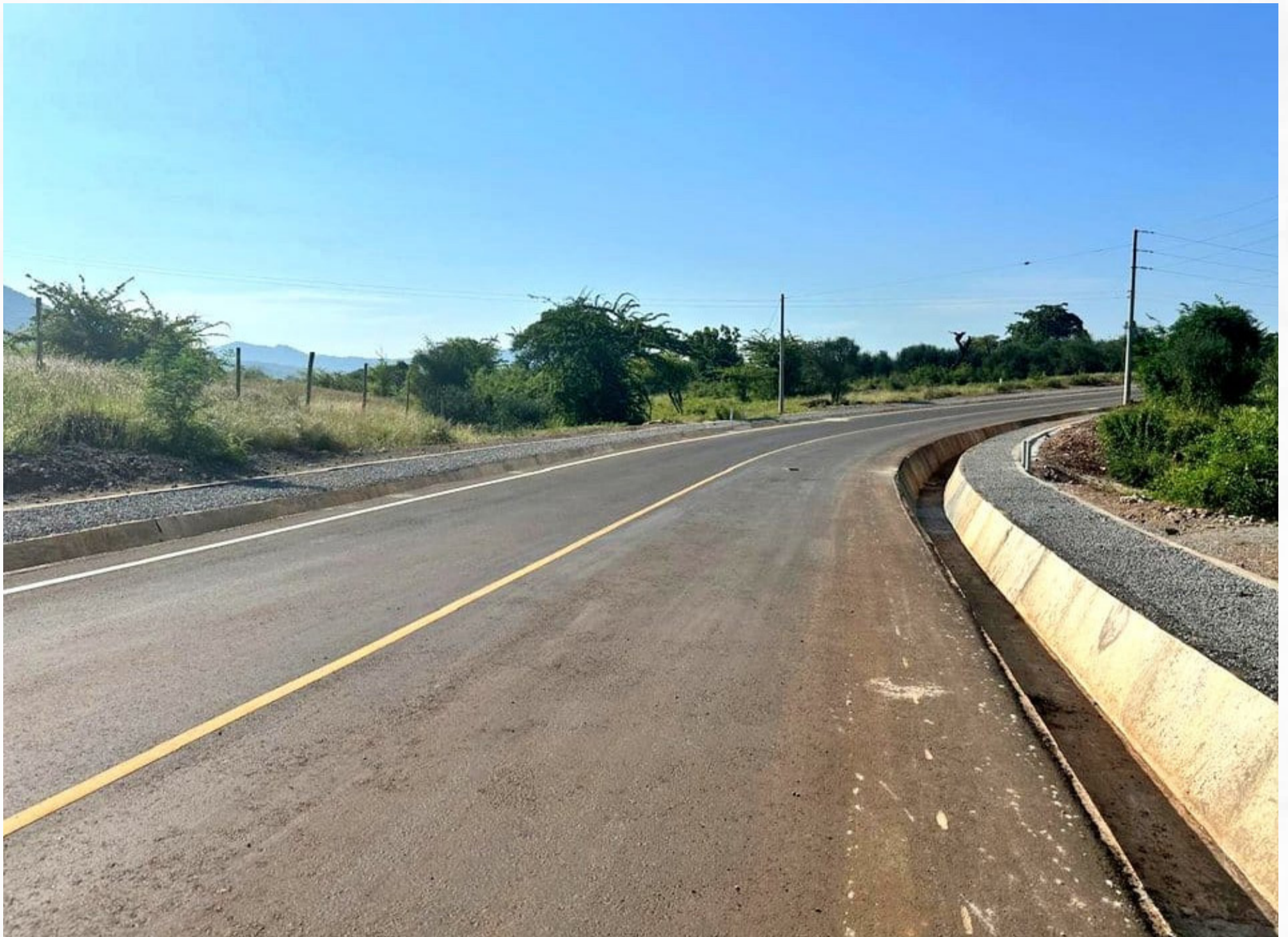
A completed section of the seven kilometres Kanjuki-Kathwana-Makutano Road in Chuka. PHOTO | KURA
