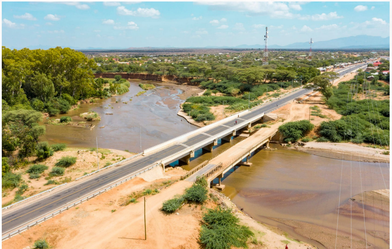
The Kainuk Bridge along the South Sudan Link Road has played a vital role in enhancing Kenya's regional integration with Northern neighbours through South Sudan. PHOTO | KeNHA
