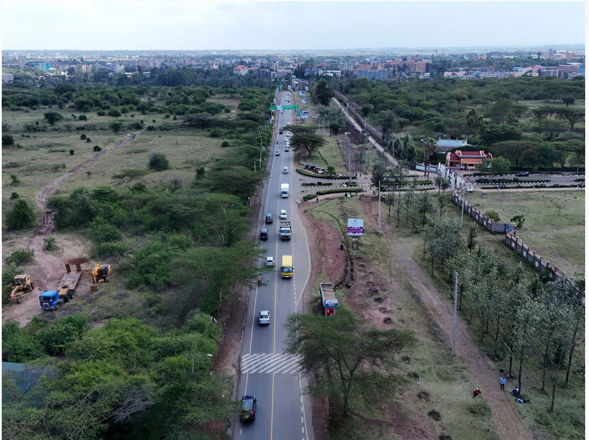
A section of the 17.5-kilometre Bomas–Kiserian (B19) Road at Multimedia University of Kenya (MMU) which cost KSh514.1 million. PHOTO | Dr Raymond Omollo, PS Interior/FB
