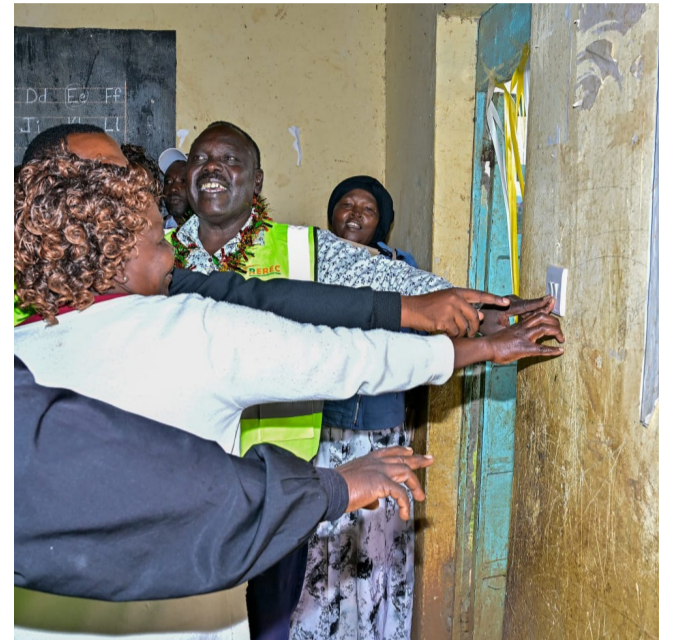
Eldama Ravine MP Musa Sirma officiated the official commissioning of the AIC Tumon Rural Electrification Project in Eldama Ravine Constituency, Baringo County. PHOTO | REREC.
