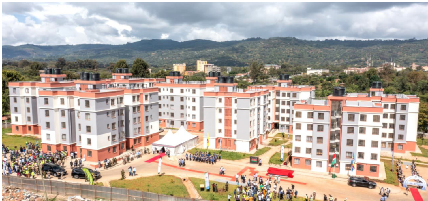
A view of the Machakos Affordable Housing projects that were handed over to beneficiaries by President William Ruto on November 14, 2025. PHOTO | PCS.
