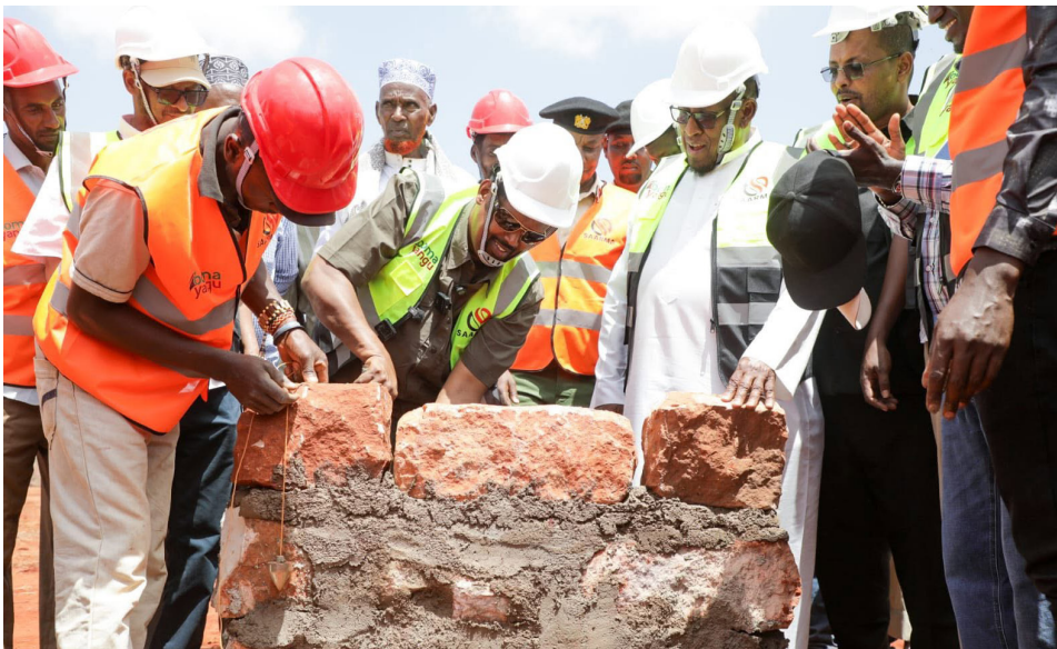
Senator Ali Roba symbolically laying the foundation stone for Takaba Technical and Vocational College (TVC) on February 9, 2026. PHOTO | Ali Roba.
