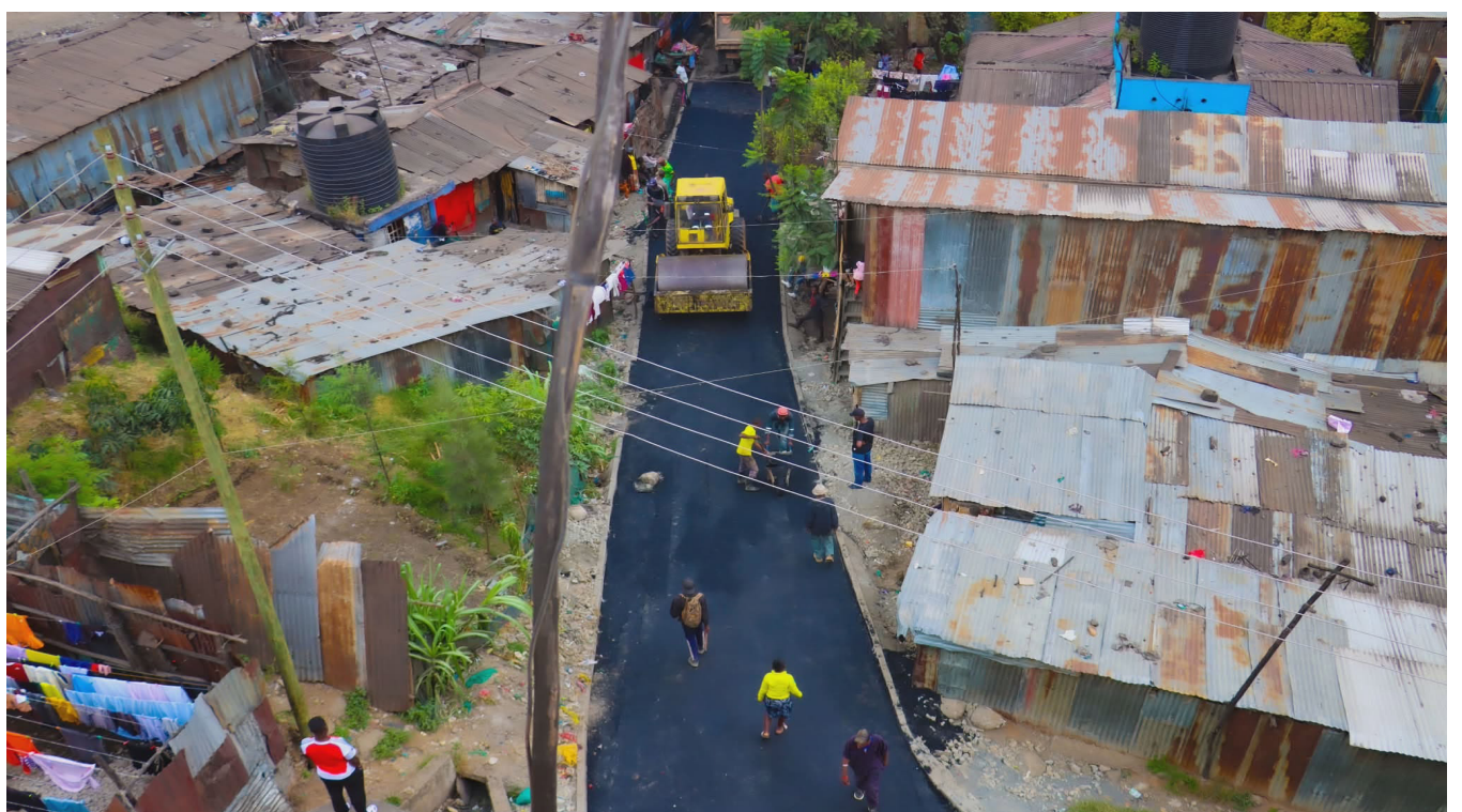
Dreams Inspiration Road connecting to Mau Mau road in June 2026. PHOTO | Hon. Wilfred Odalo
