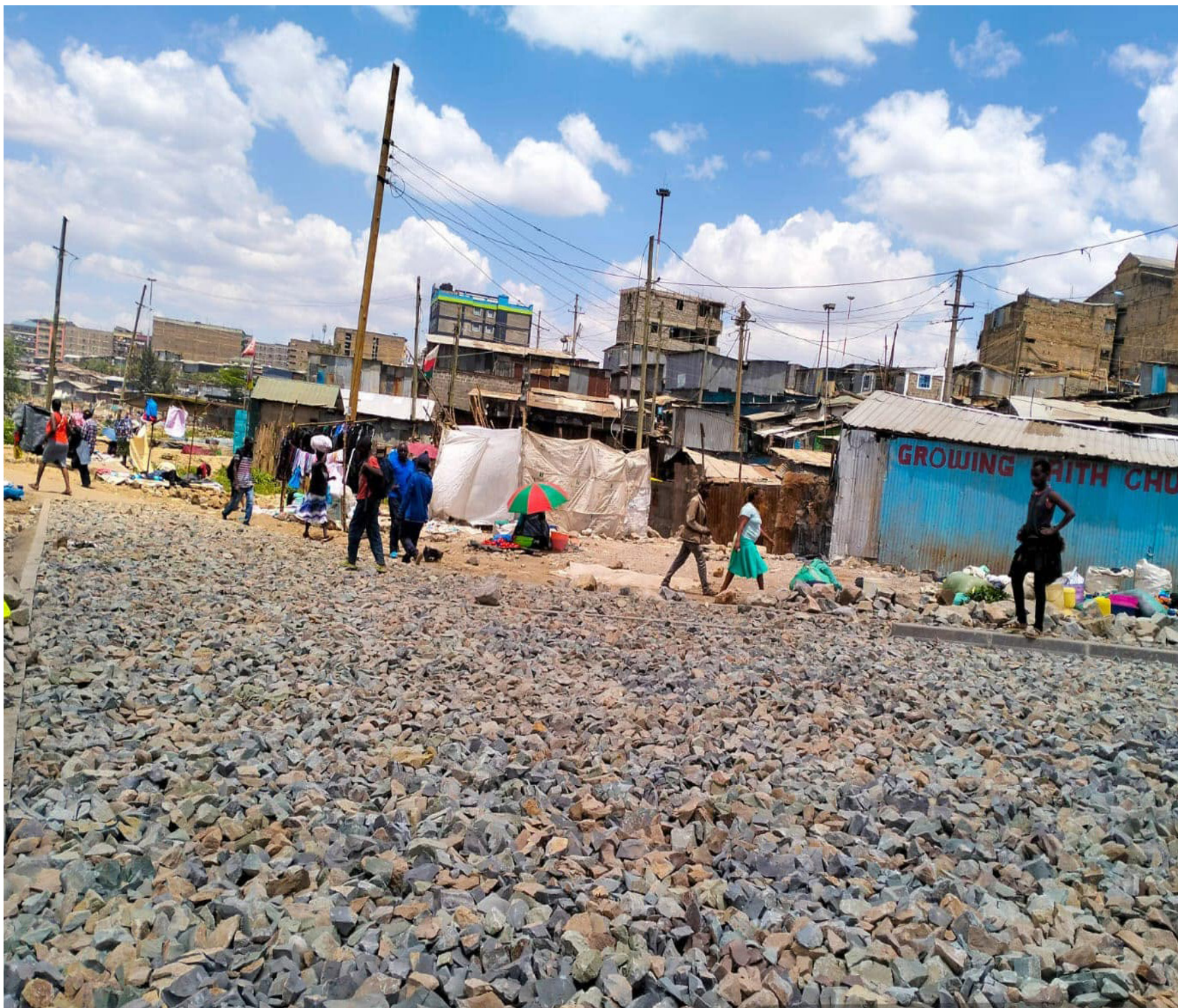
Construction of Gumba road in October 2024. PHOTO | Hon. Wilfred Odalo
