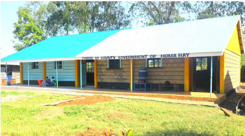
The completed Rakoro, Pala and Osure Early Years Education (EYE) classrooms in Kanyamwa Kosewe Ward, Ndihiwa Sub County. PHOTO | Homa Bay County.
