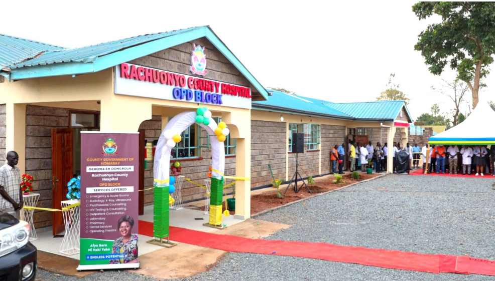
The completed Rachuoonyo South Hospital Outpatient Department (OPD) that had stalled and abandoned for years. PHOTO | Homa Bay County.
