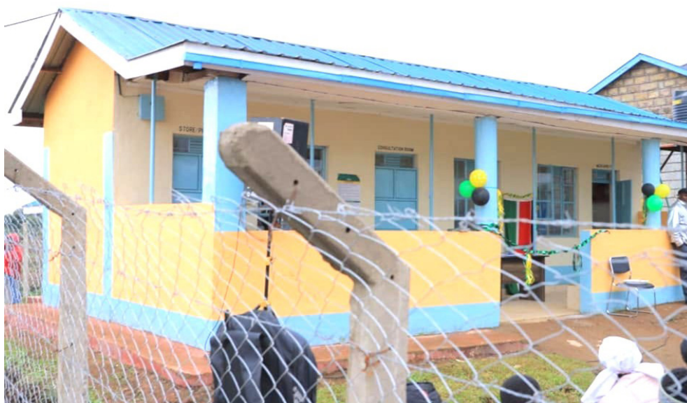
A view of Boro dispensary in Kigumo, Kinyona Ward during its official commissioning on August 25, 2024. PHOTO | Irungu Kang'ata.
