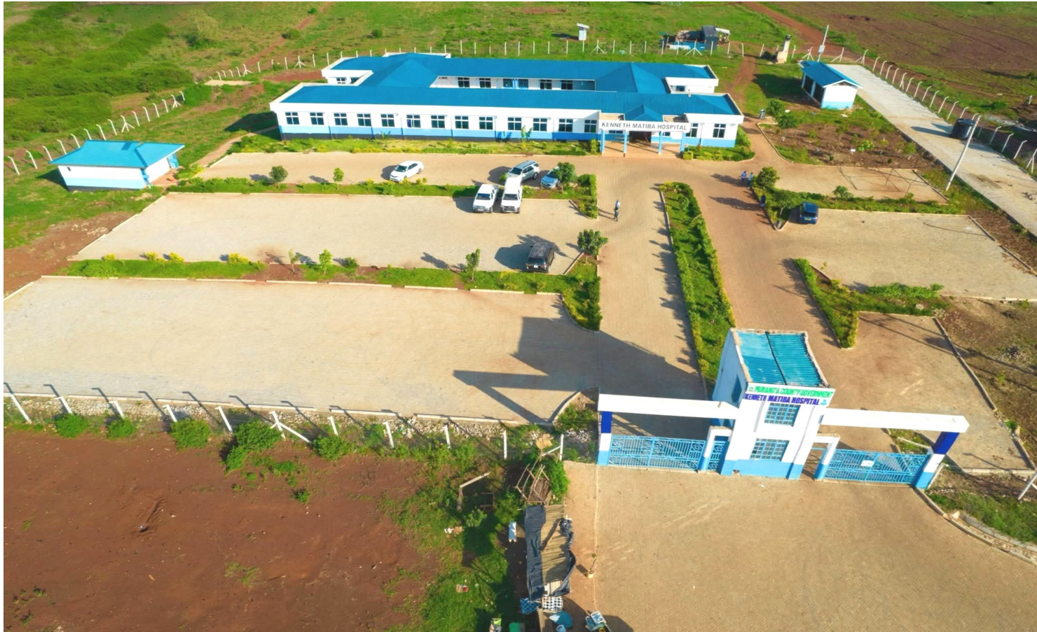
Aerial view of the Kenneth Matiba Hospital. PHOTO | Murang'a County.
