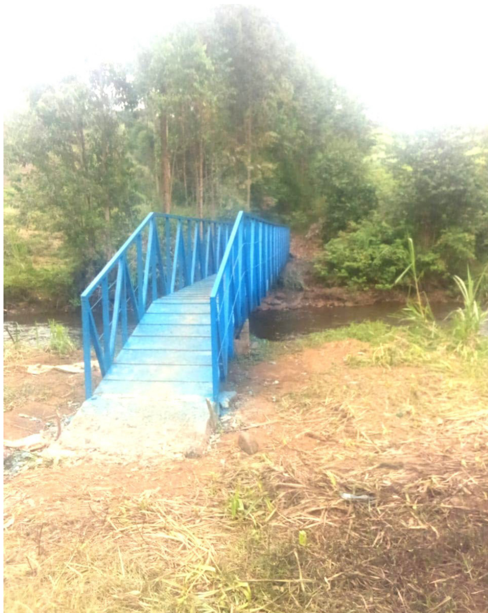
Warimwe bridge connecting Gikoe and Karinga in this July 1, 2024 photo. PHOTO | Liz Mbugua.
