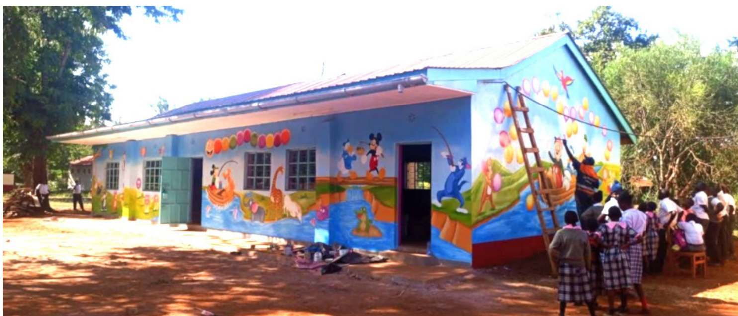
A view of Boro dispensary in Kigumo, Kinyona Ward during its official commissioning on August 25, 2024. PHOTO | Irungu Kang'ata.
