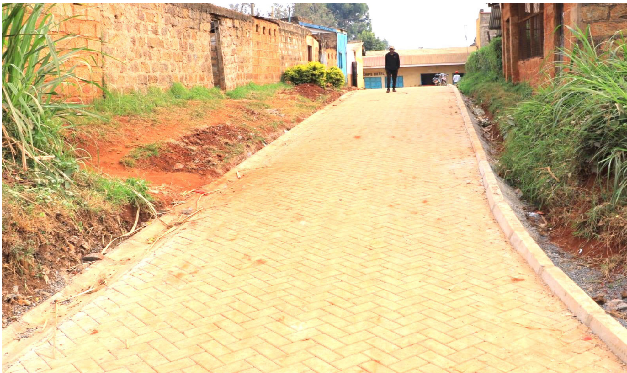
Cabro works in Mukarara that have enabled access to all businesses while creating a favourable environment during rainy seasons. PHOTO: Murang'a County.
