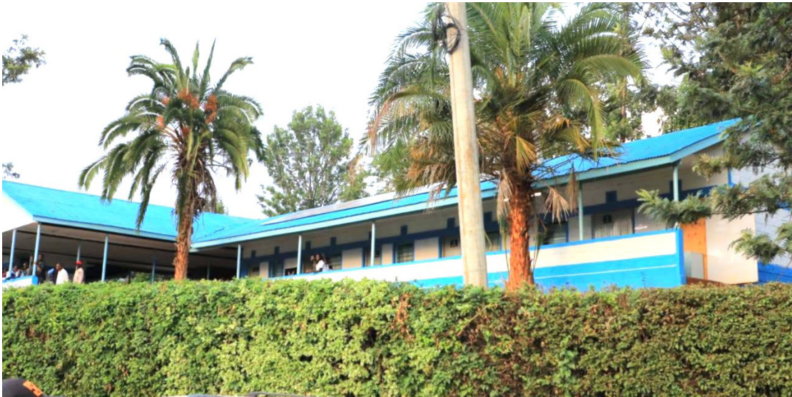
Governor Irungu Kang’ata initiated key upgrades at Sabasaba Health Centre including the installation of solar power, comprehensive renovations, an ultrasound machine and an X-ray unit. Now, the facility offers 24-hour services bringing great relief to residents. PHOTO | Murang’a County.
