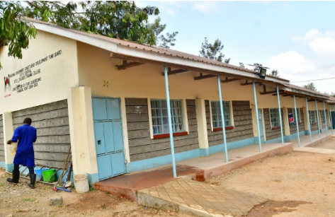
Renovated Kitui Teachers Training College. PHOTO | Milestone Badge
