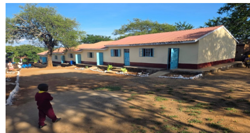
Kangundo Primary School renovated. PHOTO | Milestone Badge
