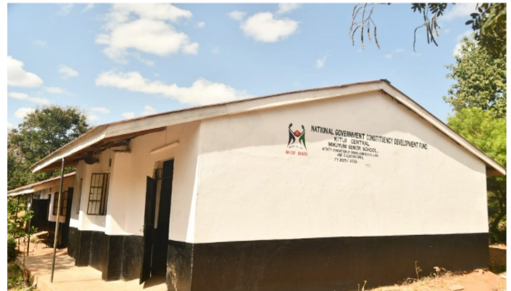
Mikuyuni Senior School's kitchen/dining hall. PHOTO | Milestone Badge
