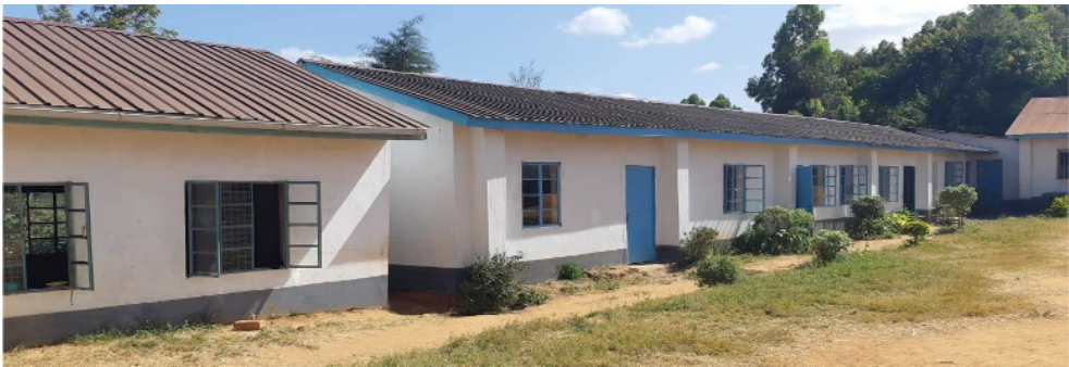
New classrooms at Mulundi Primary School. PHOTO | Milestone Badge
