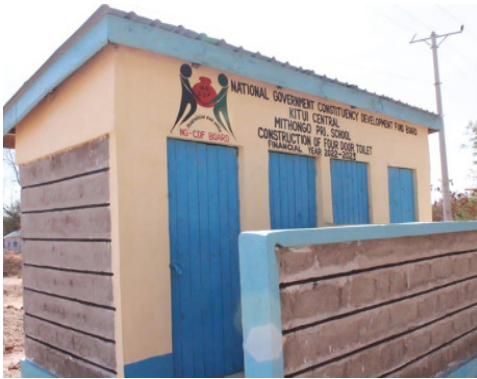
New toilet at Mithongo Primary School. PHOTO | Milestone Badge
