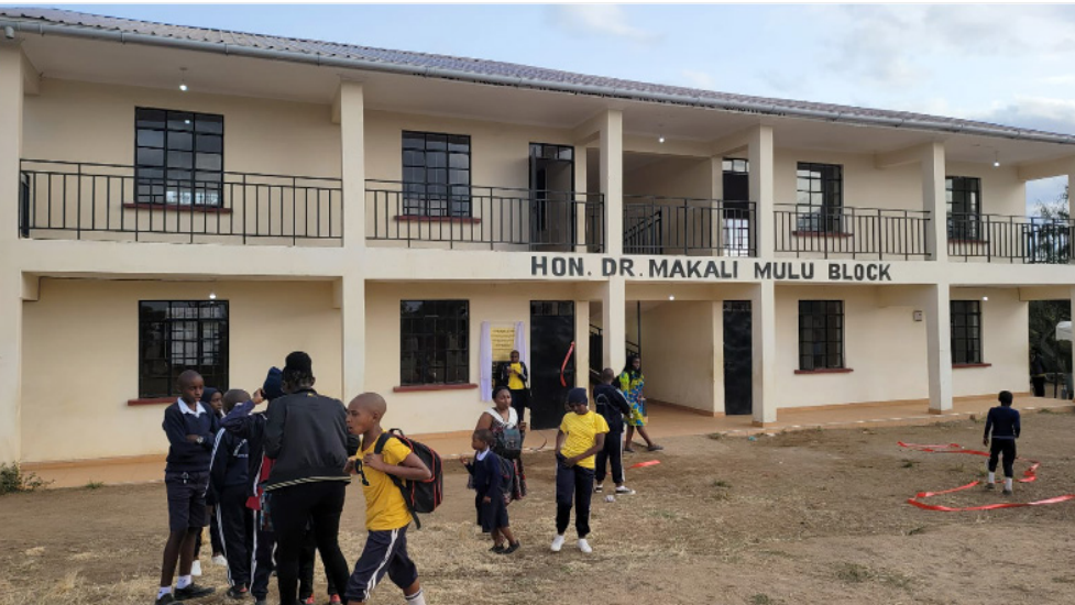
New classrooms at Unyaa Primary School. PHOTO | Milestone Badge
