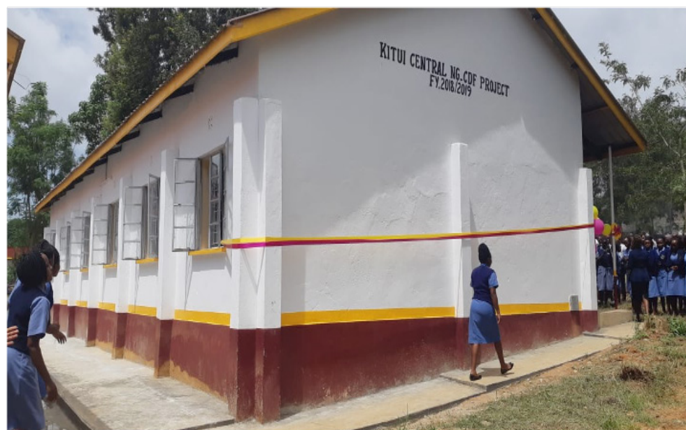
Kitui KMTC lecture hall. PHOTO | Milestone Badge
