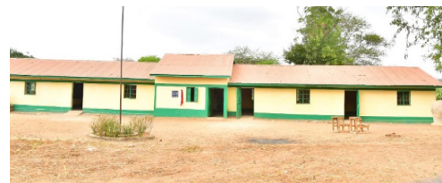
Ivovoa Primary School block of classrooms renovated. PHOTO | Milestone Badge
