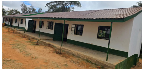
Wanzua Primary School renovated. PHOTO | Milestone Badge
