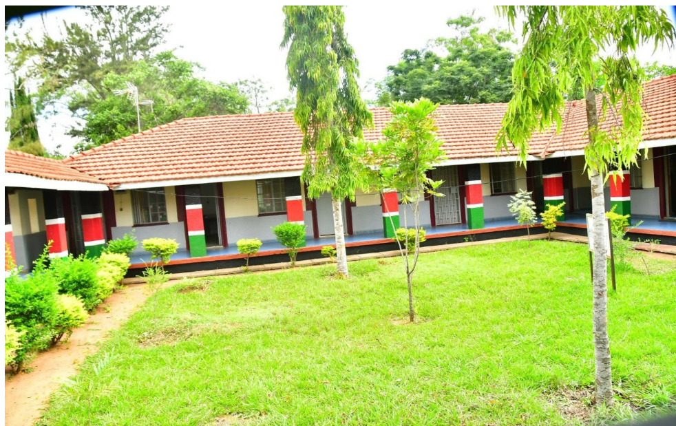
The newly renovated Deputy County Commissioner's office. It was commissioned by Hon. Dr. Makali Mulu on January 23, 2026. PHOTO | Milestone Badge
