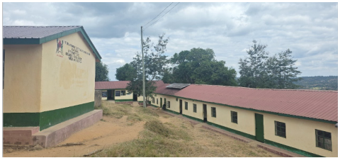
Katia Primary School block of classrooms renovated. PHOTO | Milestone Badge
