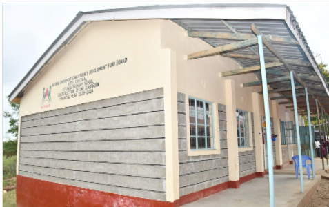
Kitundu Primary School's new JSS classroom. PHOTO | Milestone Badge
