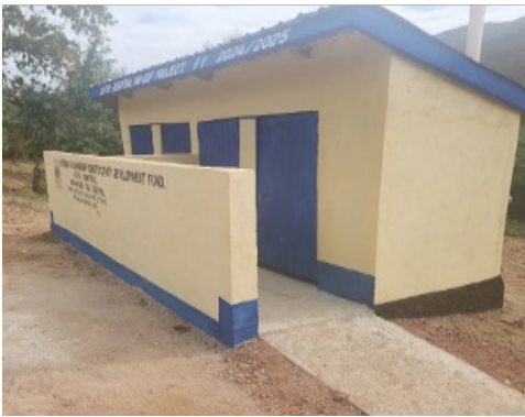
Exhaustible toilet at Mikuyuni Secondary School. PHOTO | Milestone Badge
